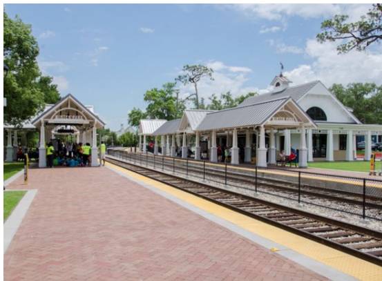
Figure 8.5d: Example Commuter Rail Station
